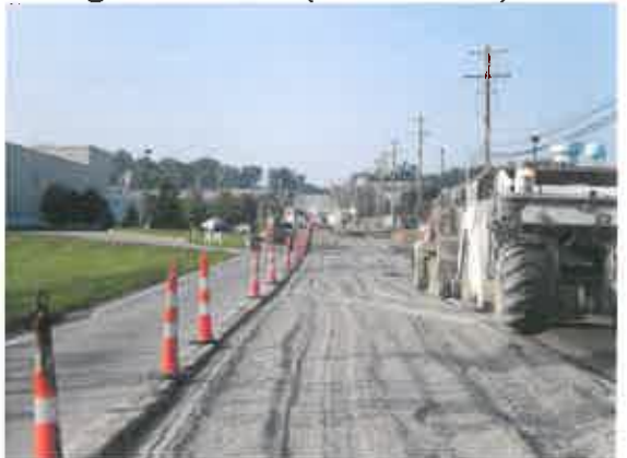
During Construction (Seward Road):
